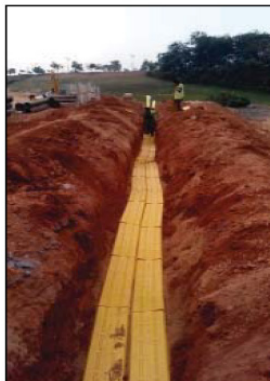
Laying of Protection Cover for gas pipe
