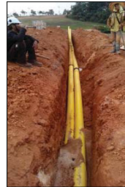
Laying of Gas Pipe
